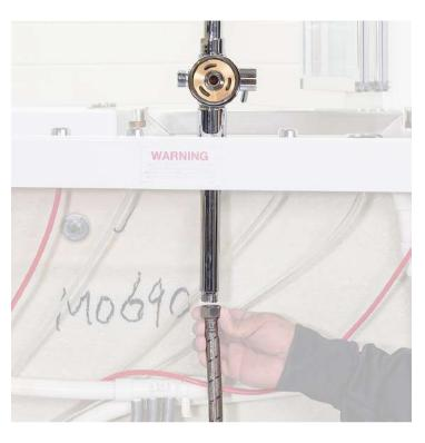
Tighten supply hose on the bottom of shower column
